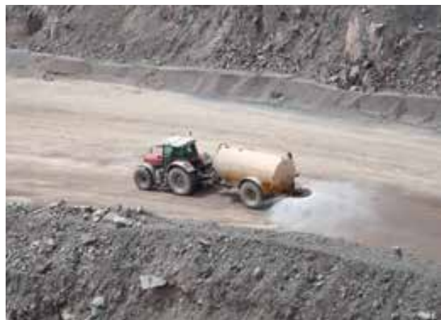
Figure 2 - water sprays on dusty road
